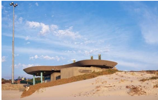
1970 Floreat Beach Kiosk, one of three off form concrete kiosks (Fabric Quarterly 09 2017).
